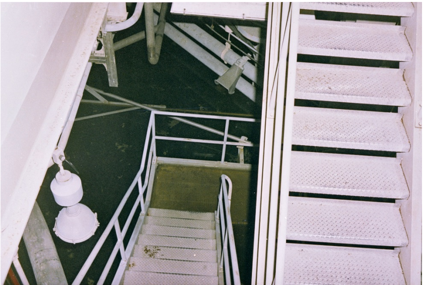
Water level in the reactor building basement reached the first stairwell landing, indicating about 8 feet of water. The submerged demineralizer system or “SDS” was designed and installed to cleanup the 700,000 gallons of highly contaminated basement water. The SDS started operations in September 1981 after NRC approval and completed processing basement water in May 1982.
